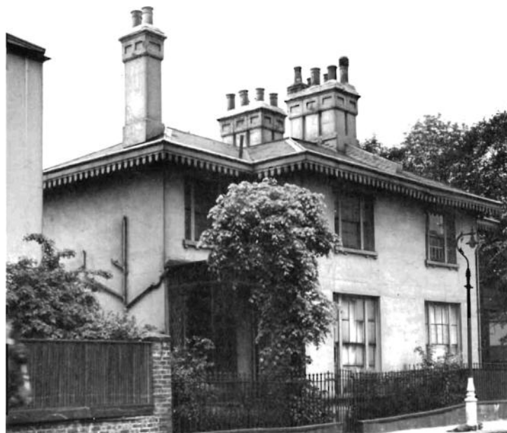
5 Double Cottage, Park Village East, Regent's Park, Londres, Angleterre; Construction en 1824; John Nash, architecte; revêtement: stuc.
